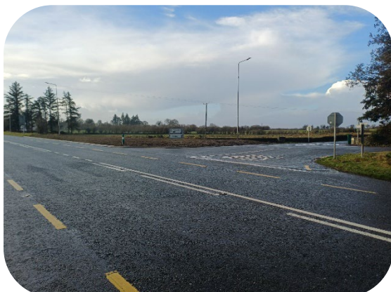
N17 - L 8319 Curry Road Safety Improvement Scheme
